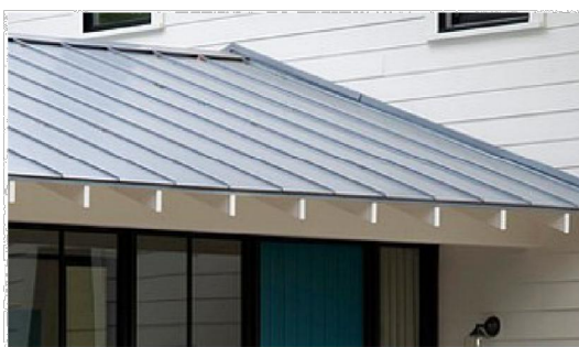
EXPOSED EAVES WITH BEAM TAILS (2 FT OVERHANG & GREATER OVERHANG)
